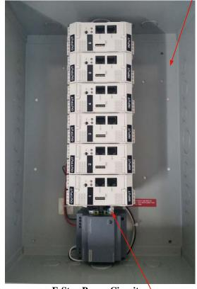
**E-Stop Power Circuit** supplies 120VAC power source to the DED Combo panel.
